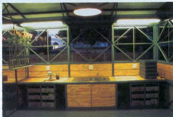
Above right: Additional steel was purchased for the roof purlins and bracing, and to construct the frames for work surfaces, shelving and drawer units in the studio. The steel float-screeded floor slab is finished with floor enamel.
